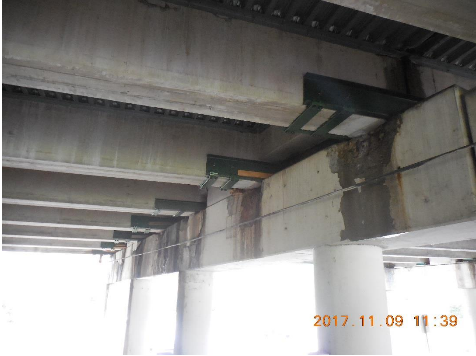
Looking at Bent and Beam Supports
