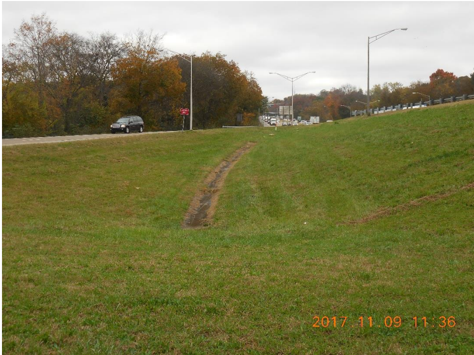
Drain at Southwest side of Bridge
