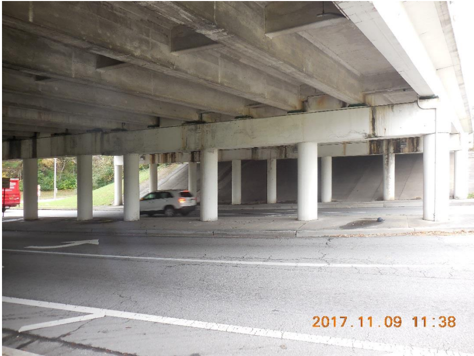
Looking under Bridge at Bents
