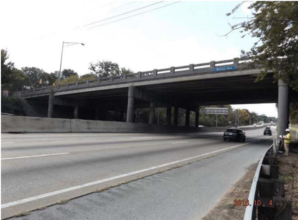
Bottom of Deck / Clearance – Westbound (Right Side)
