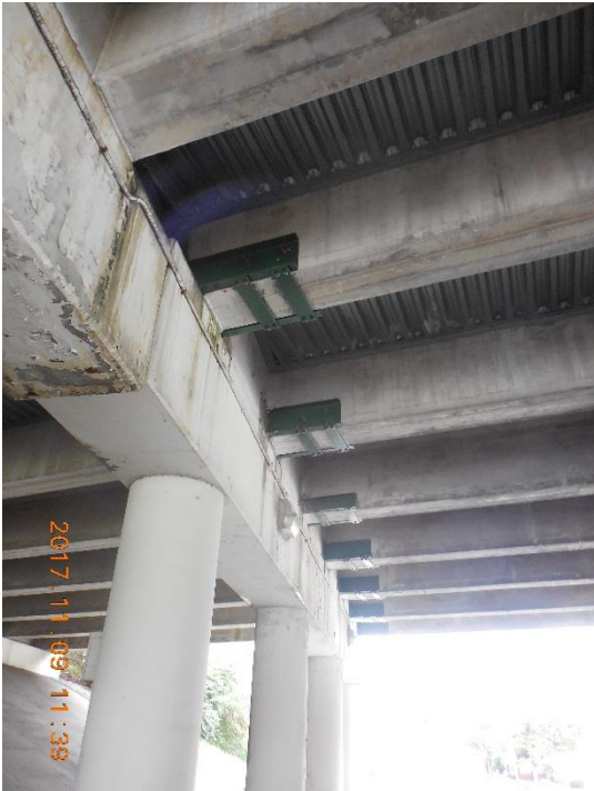
Looking at Underside of Deck
