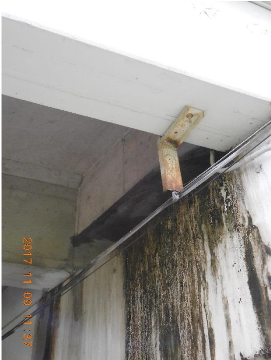
Utilities Mounted to Bridge
