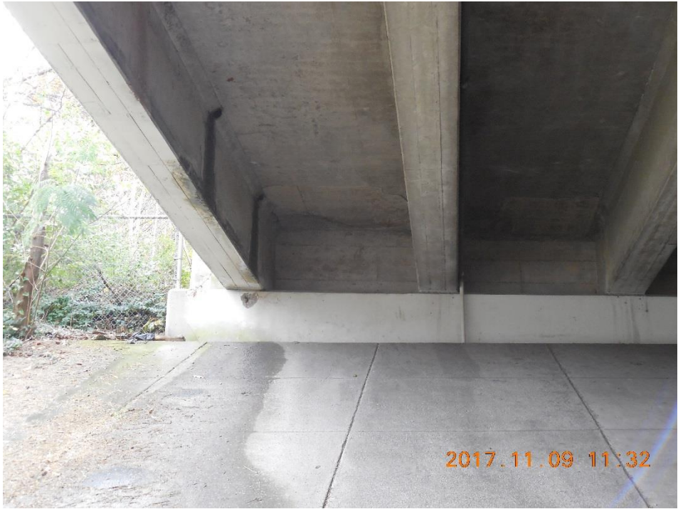
Looking at Abutment No. 2
