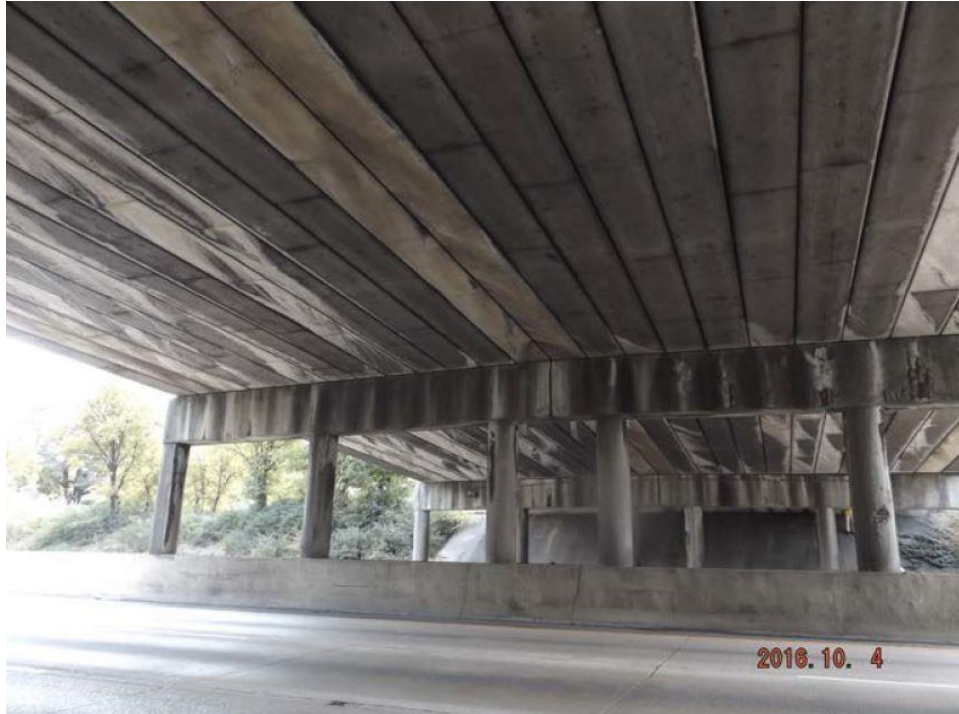
Span No. 3 / Bent No. 2
