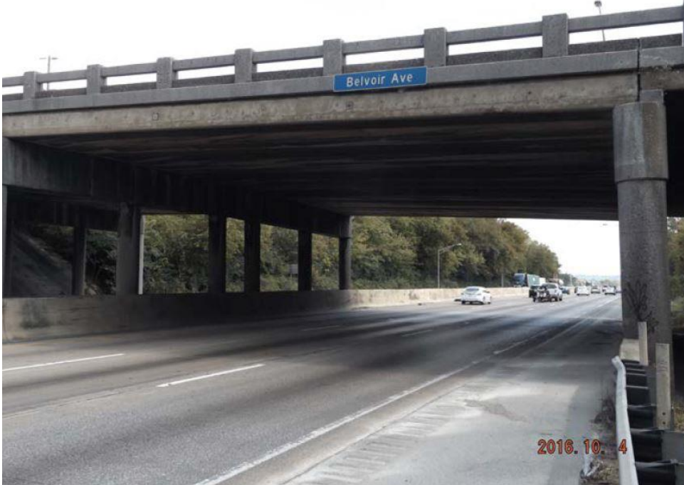
Bottom of Deck / Clearance - Eastbound
