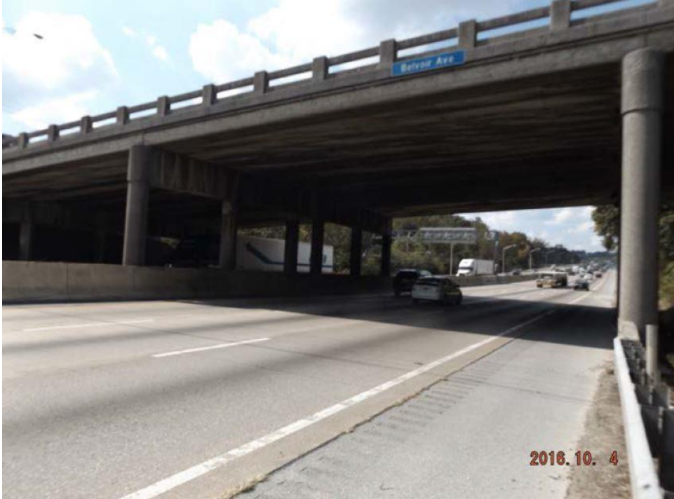
Bottom of Deck / Clearance – Westbound
