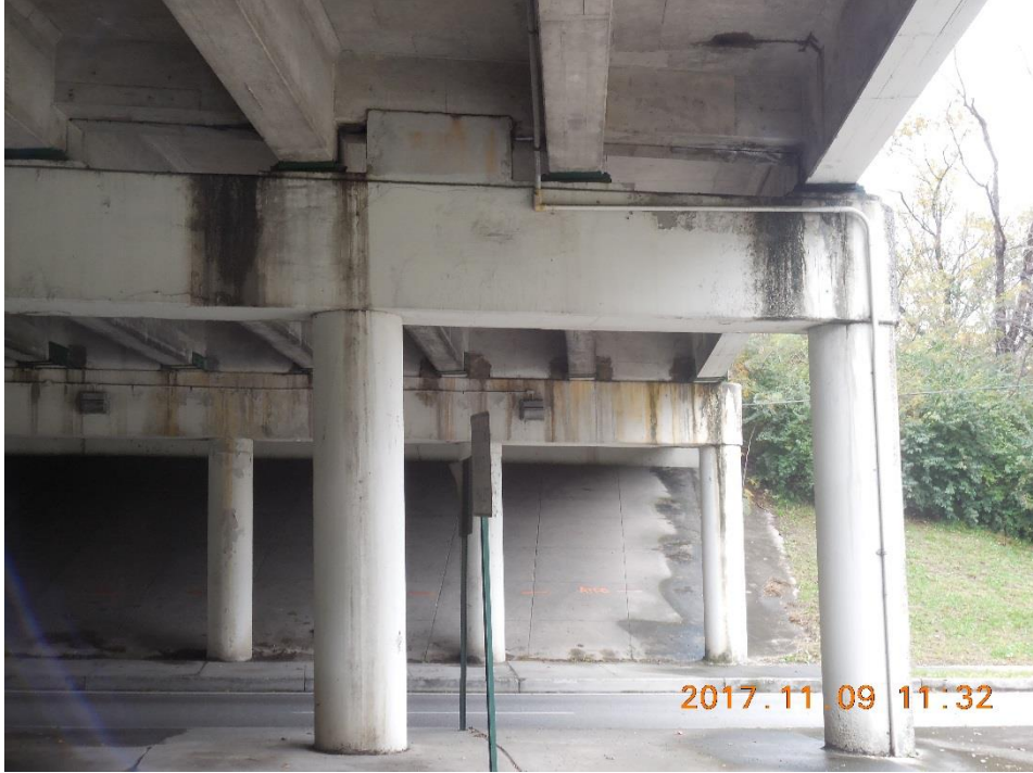
Looking at Bents No. 1 and No. 2
