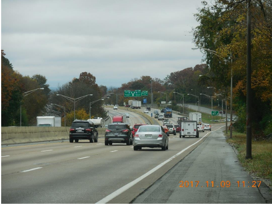
Looking East over Bridge
