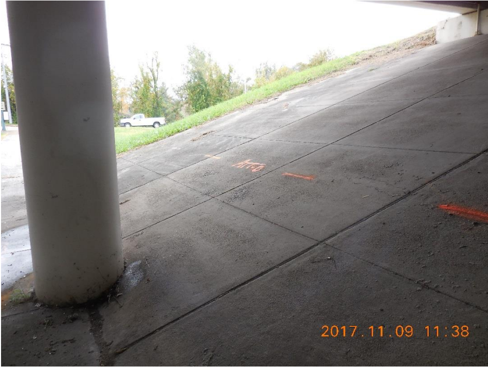
Concrete Slope Paving
