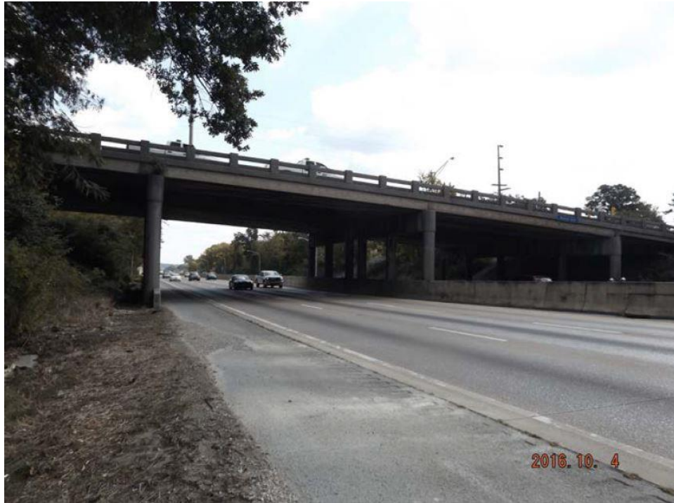
Bottom of Deck / Clearance – Westbound (Left Side)
