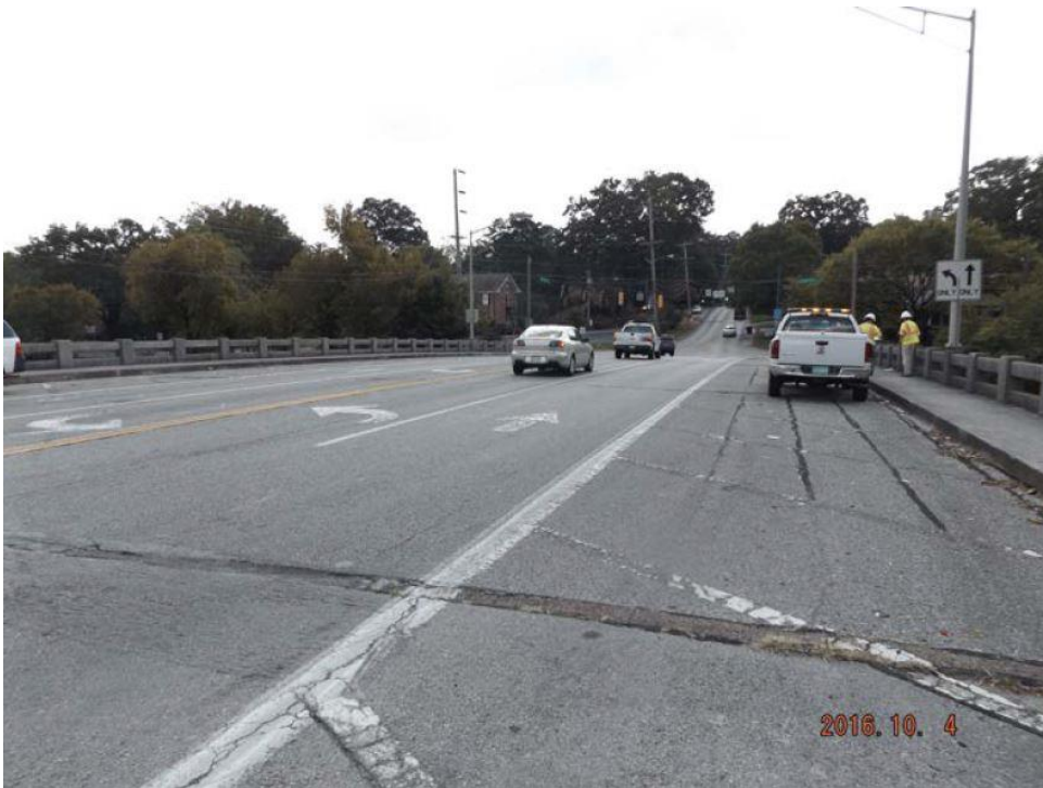
Top of Deck - Southbound
