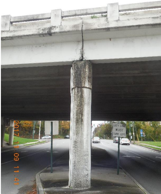
Looking North at Bent No. 2
