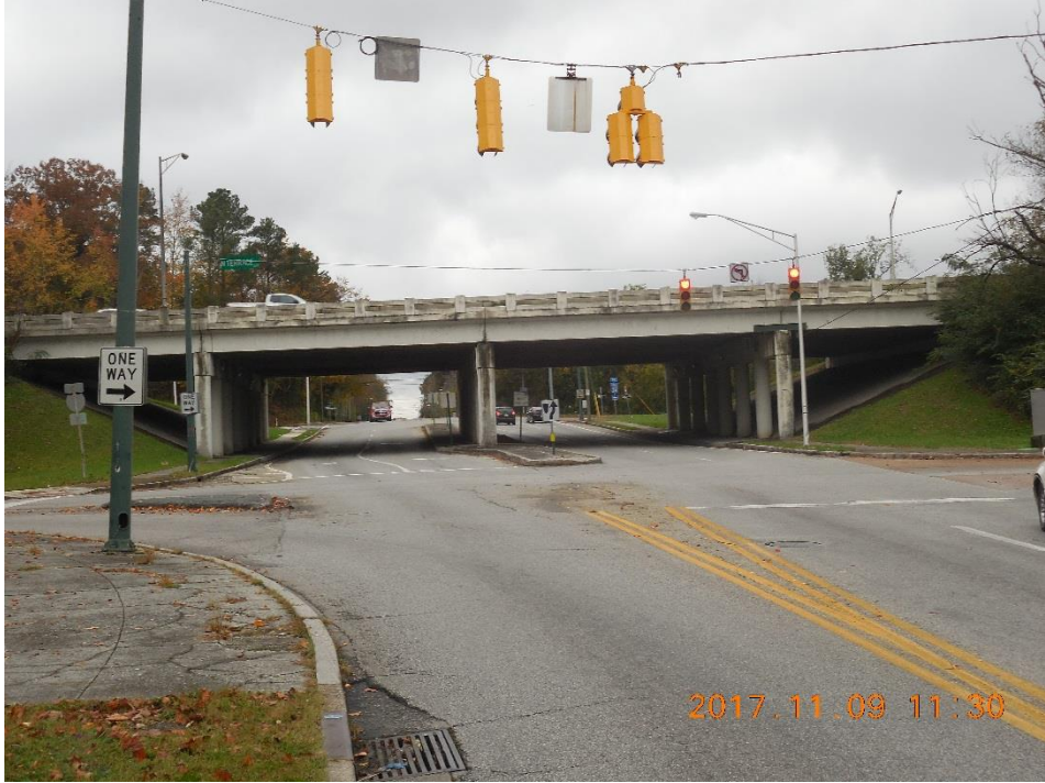
Looking South under Bridge
