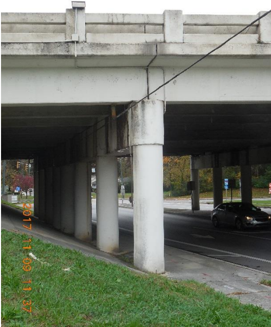
Looking at Bent No. 1
