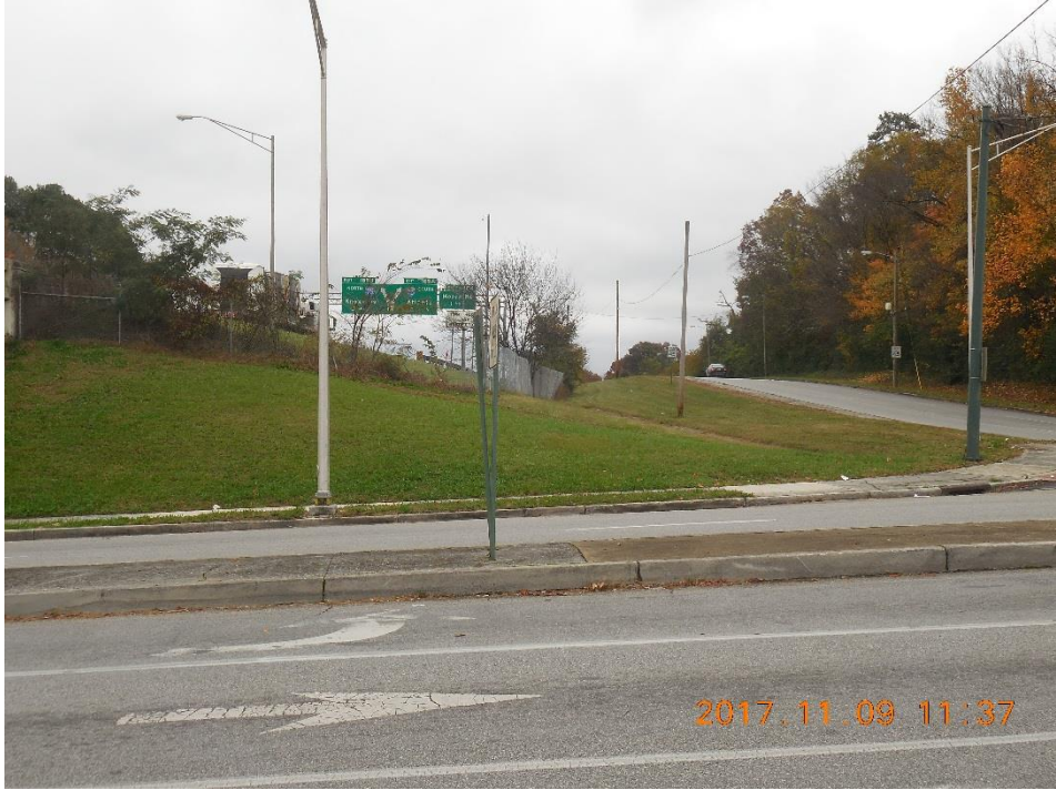
Looking East at On-Ramp
