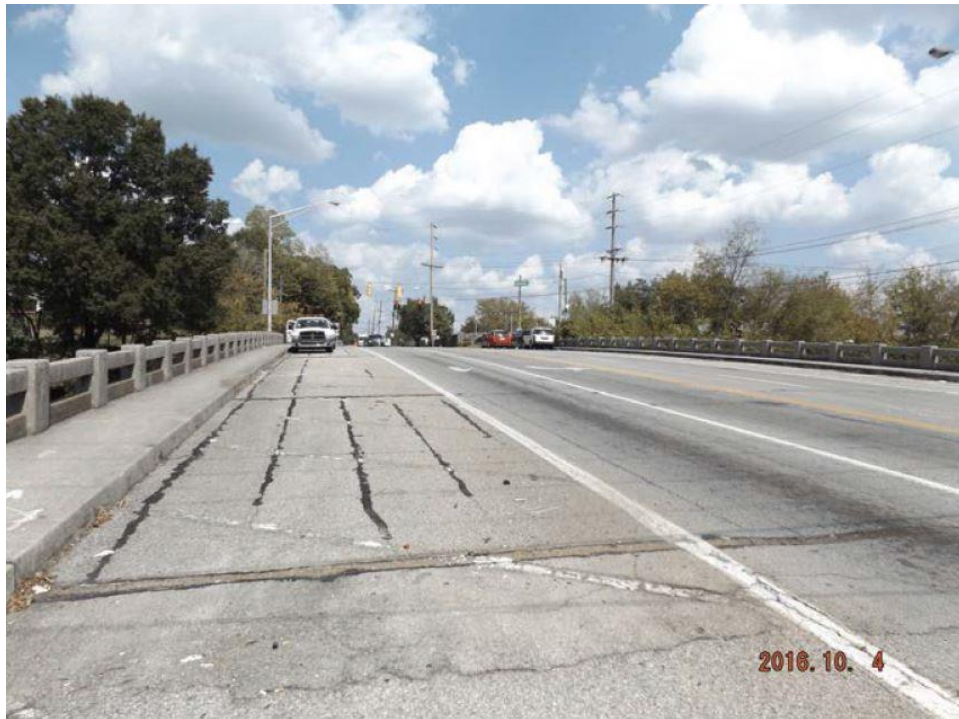
Top of Deck - Northbound
