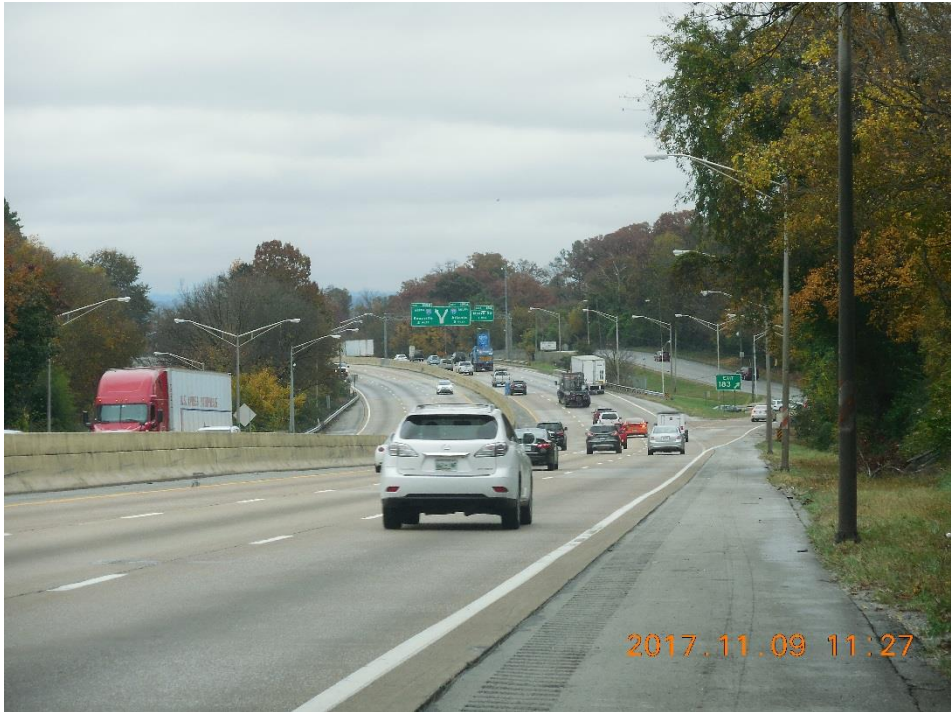
Looking East over Bridge
