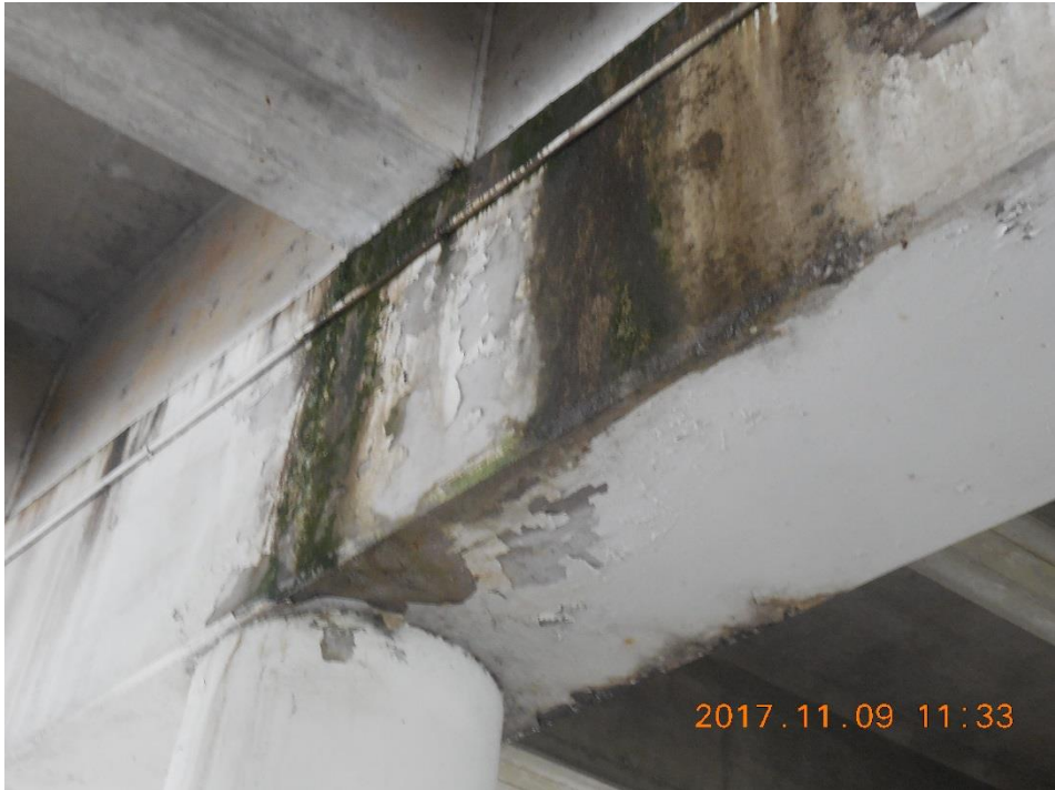
Underside of Bent Cap
