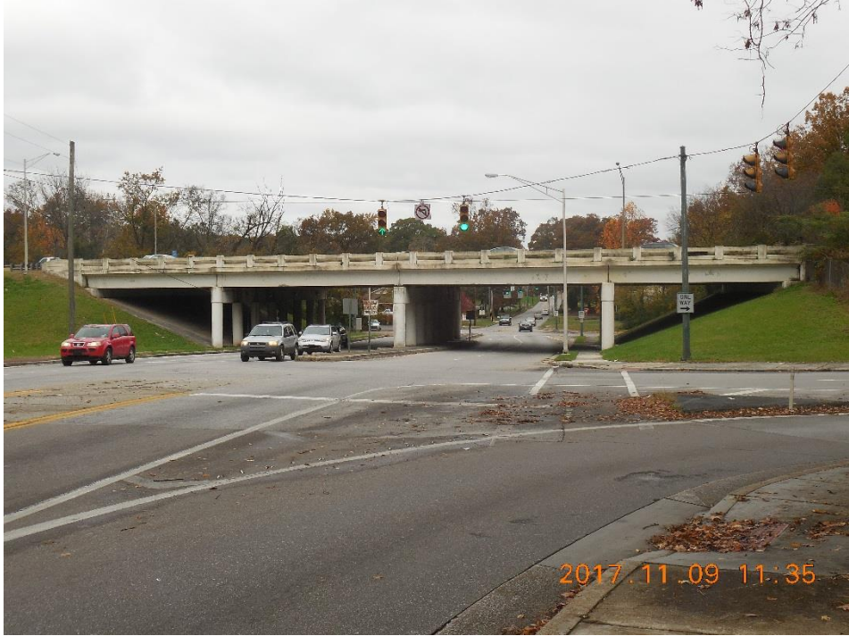
Looking North under the Bridge
