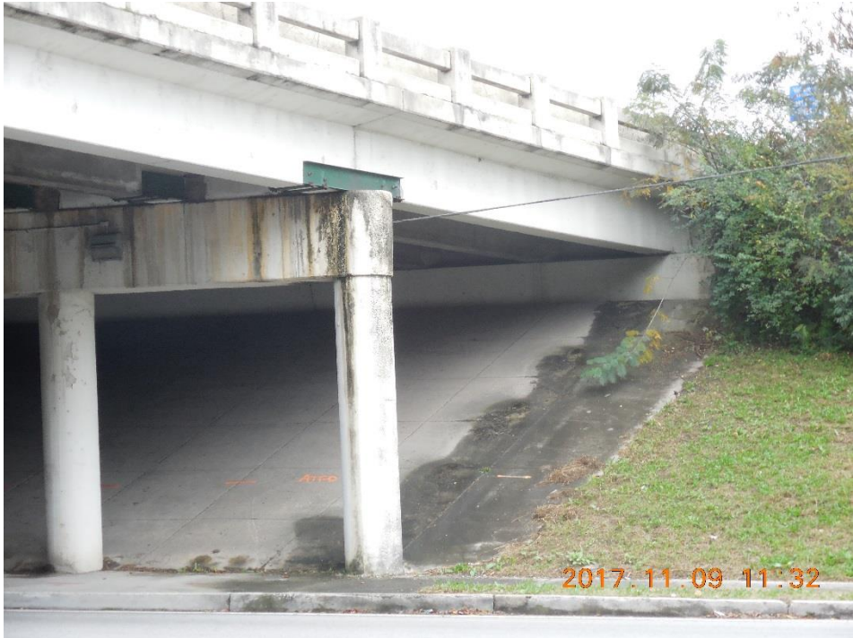
Looking at Abutment No. 1
