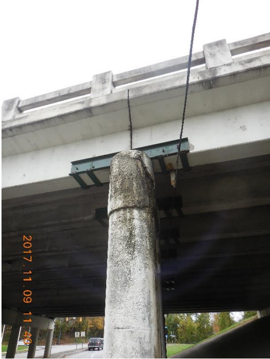
Looking at North at Bent No. 3
