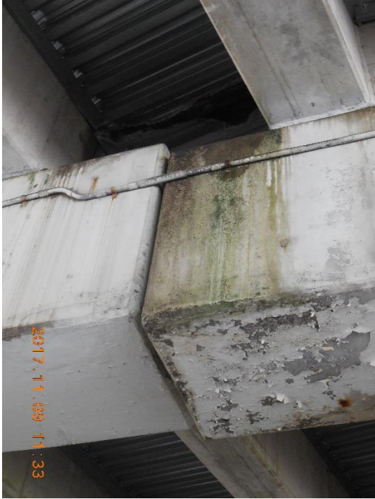
Widened Bent Caps
